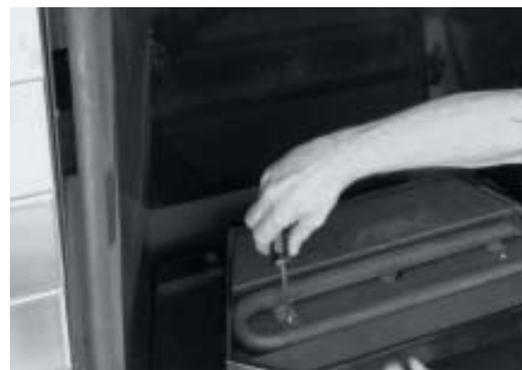
BURNER INSTALLATION
