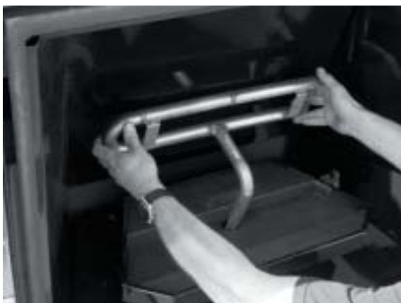
BURNER INSTALLATION
