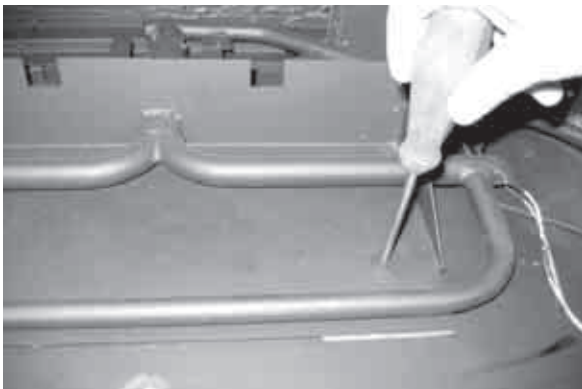
BURNER TRAY INSTALLATION
