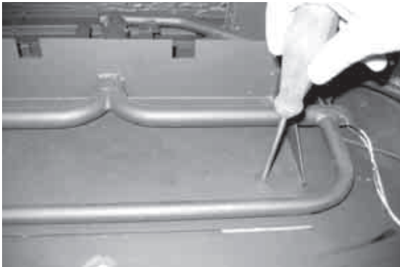
BURNER TRAY INSTALLATION
