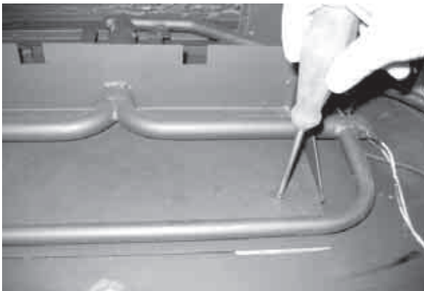
BURNER TRAY INSTALLATION
