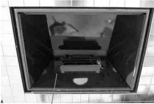
INSTALLING BURNER SHIELD
