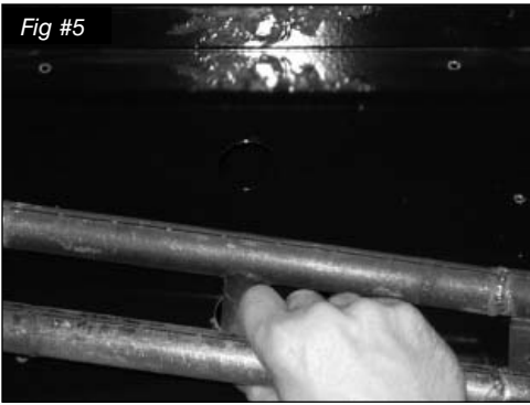
INSTALLING FRONT BURNER
