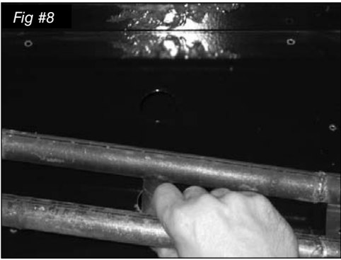
INSTALLING FRONT BURNER
