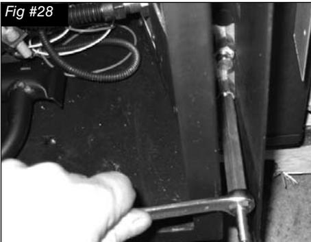
2. Thread the extension test fitting into the open test port. (Fig. #28)
