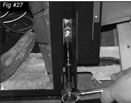
1. Remove the plug from the pressure test port using a 7/16" socket and extension. The plug is located between the right side lintel and firebox side. (Fig. #27)
