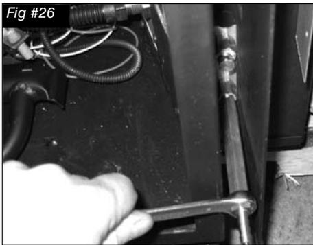
2. Thread the extension test fitting into the open test port. (Fig. #26)
