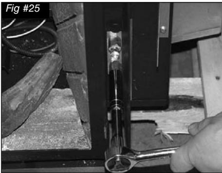
1. Remove the plug from the pressure test port using a 7/16" socket and extension. The plug is located between the right side lintel and firebox side. (Fig. #25)
